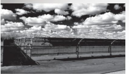
Construction and installation of the Medicine Hat Solar Thermal Plant; the first of its kind in Canada and one of only a few in the world. Dynamic Industrial Solutions fabricated the 5.56 acre plot of curved steel panels that reflect the sun's rays to heat oil inside a metal tube. The oil then creates steam, turning a turbine at the nearby power plant.
